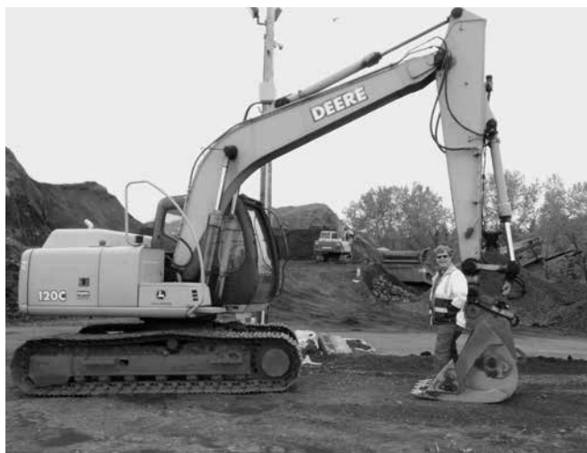
Environmental Services - Hartwell Ave
