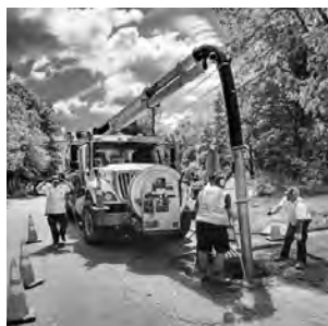
Highway Division: storm drain maintenance.
