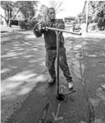
Water and Sewer: main shut-off valve.
