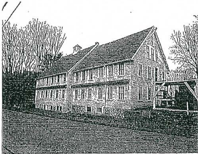
BARN (December 14, 2011 - Photographer Kenneth Croft)
