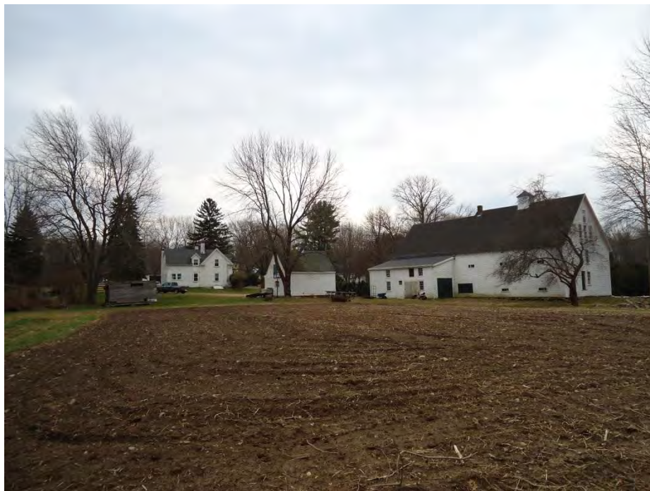
REAR OF BARN GARAGE & HOUSE (December 14, 2011 – Photographer Kenneth Croft) SUBJECT PHOTOGRAPHS
