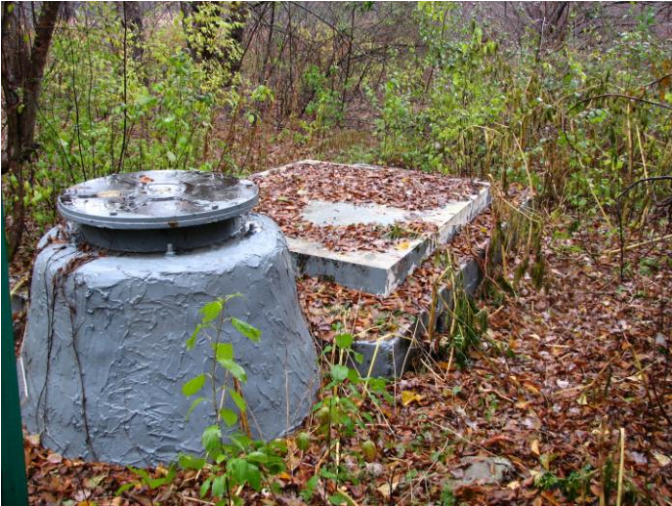
Photo 1. Sewer alongside trail. Mowed access should be maintained.
