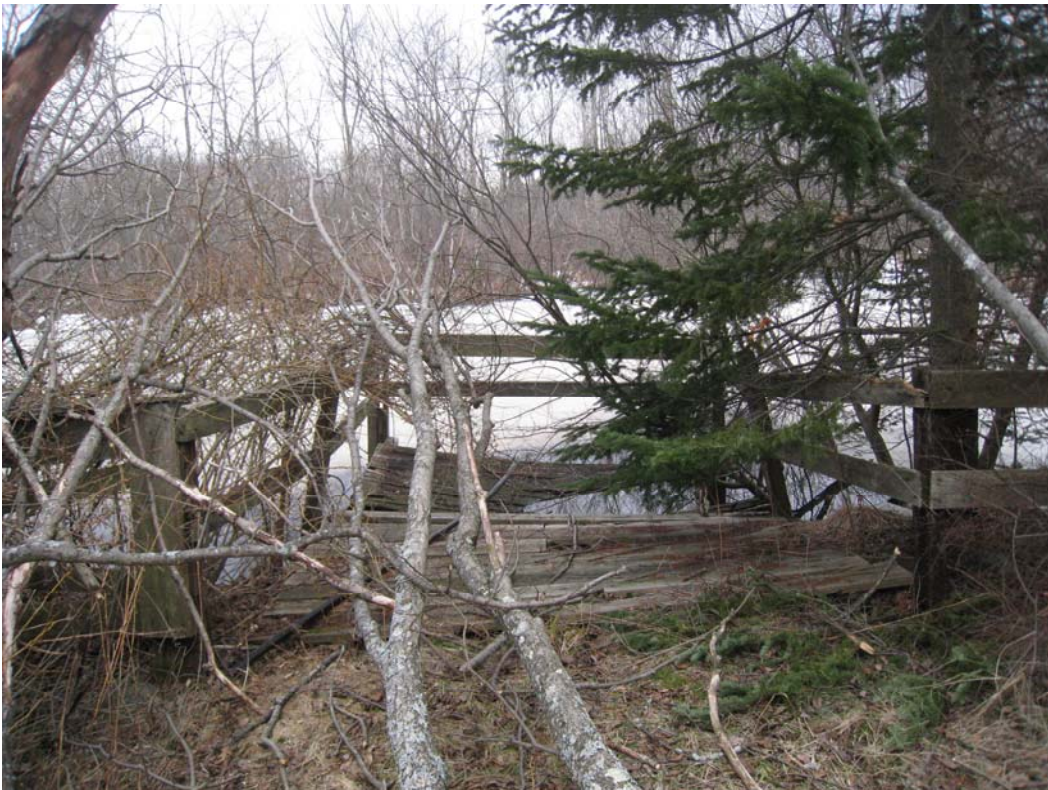
18. Dock (to be removed) at the pond edge
