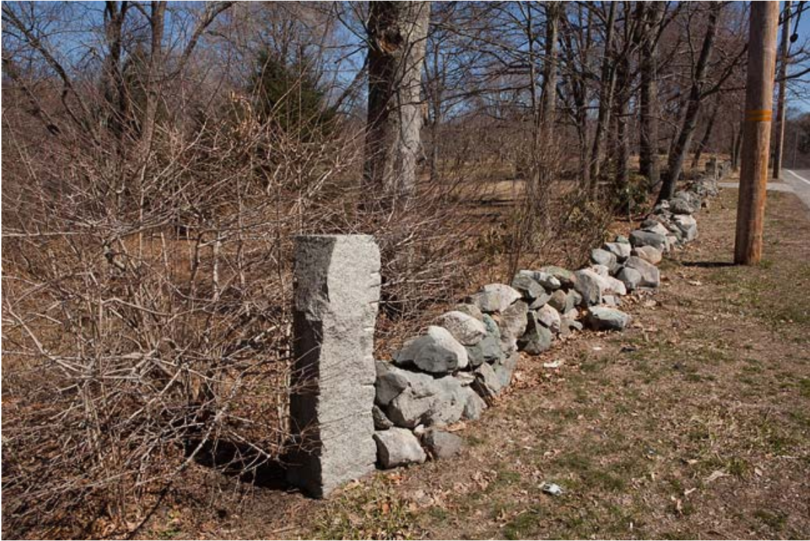
1. SW Corner, looking east along Marrett Road
