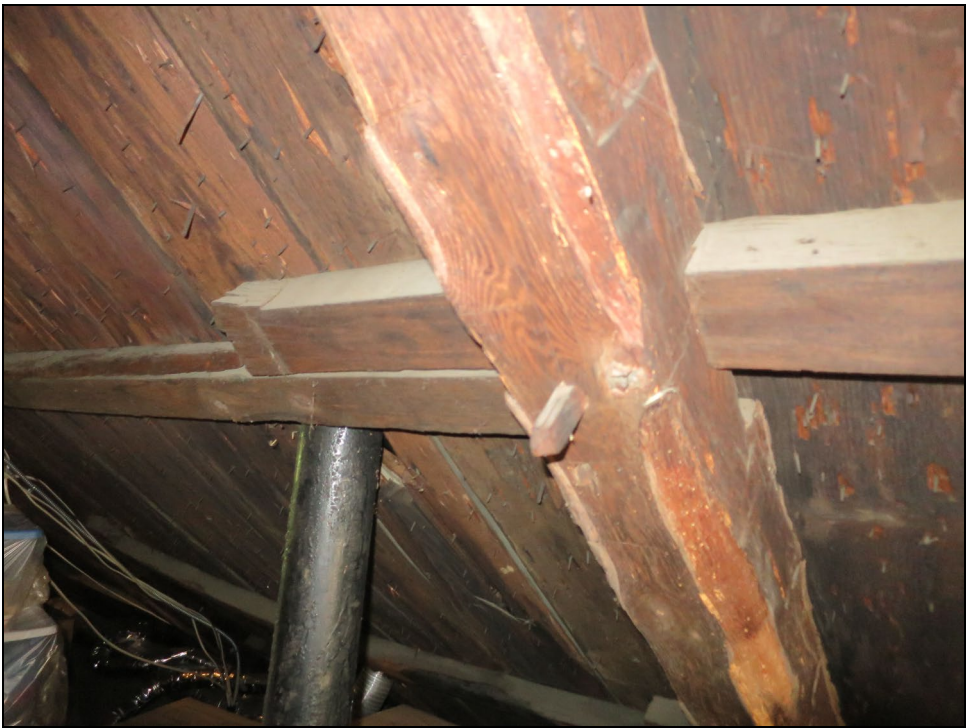
Attic, detail of principal rafter and common purlin joinery.
