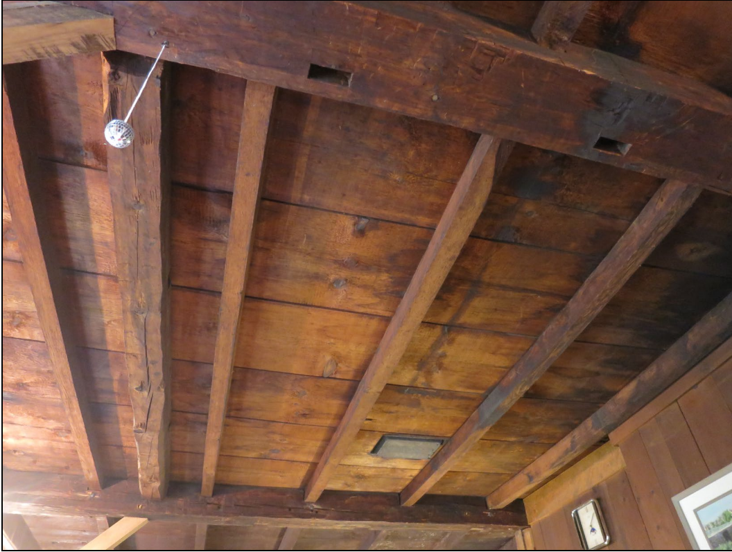
Kitchen wing, first floor, framing in ceiling showing beam with mortises for dividing wall.
