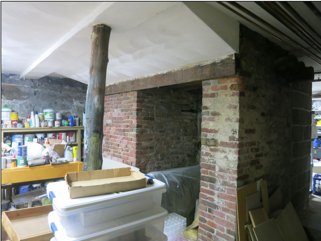
Kitchen wing, basement, chimney base for cooking hearth.
