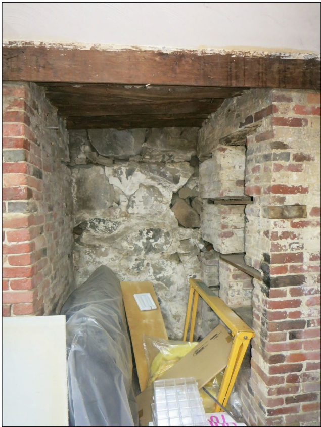
Basement, detail of brick base for west chimney.
