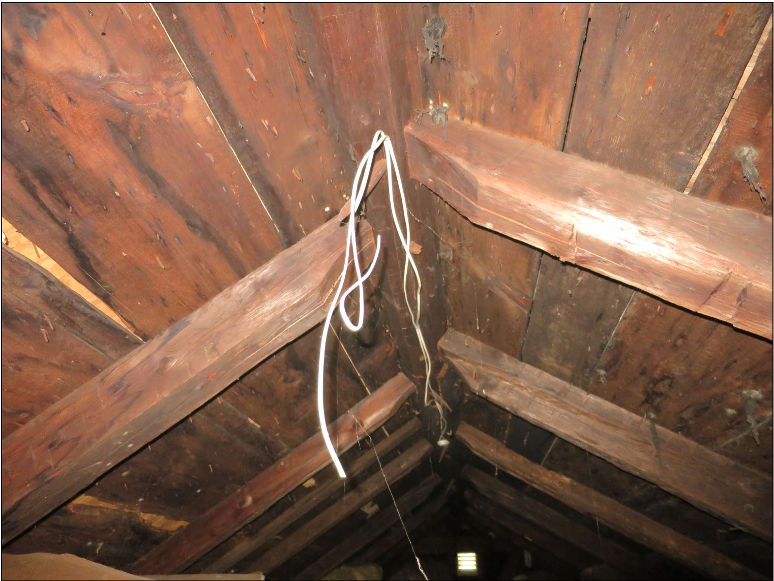
Kitchen wing, attic, view of rafters, ridge pole and joinery method.
