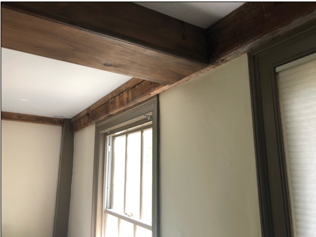
Second floor, SE chamber showing corner posts, girts and summer beam exposed when original plaster ceiling was removed. Summer beam now cased.
