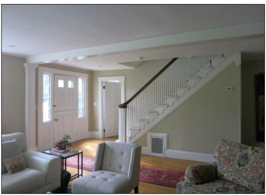
Living room with entry and stairs in ca. 1895 renovation of store section looking NW. Note ceiling beam for absent hall partition.
