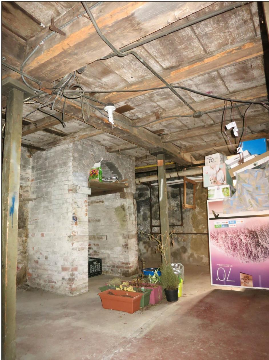
Addition basement showing arched base of front chimney and intact floor framing.
