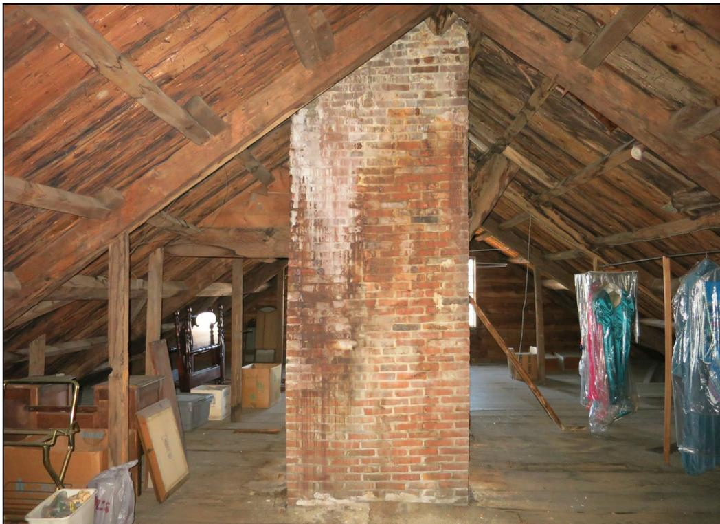
Roof framing and center chimney looking north.
