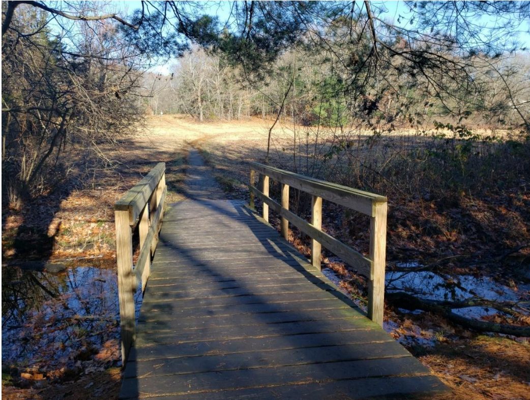
View looking northeast across footbridge towards North St. entrance.
