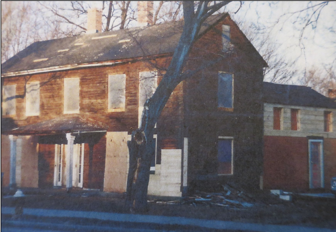
View from SW during renovation. Owner's collection.
