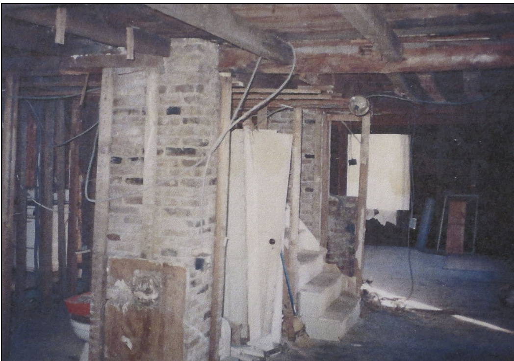
Looking south from north parlor during renovation. Owner's collection.
