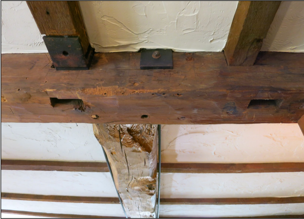
First floor, partition beam between south parlor and wing.
