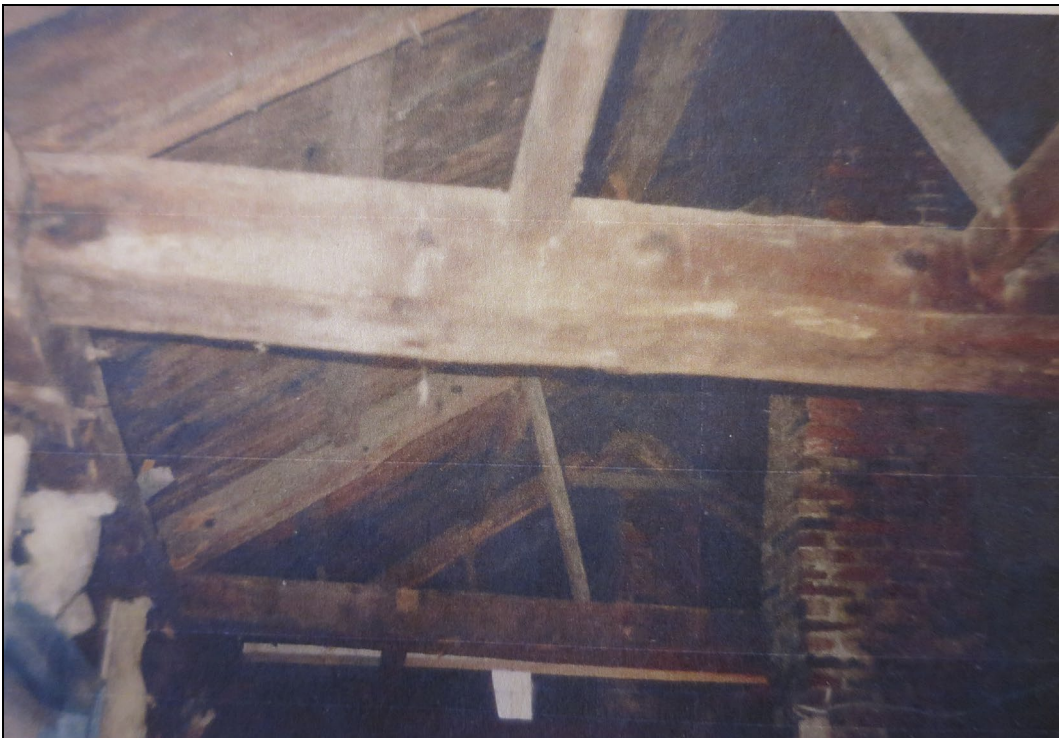
Roof framing. Owner's collection.
