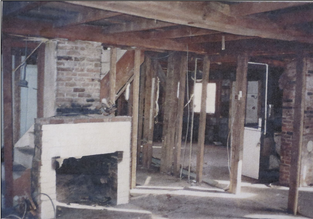
South parlor looking north during renovation. Owner's collection.
