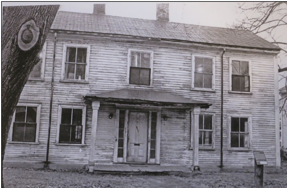
View of house before renovation in 1988. Owner's collection.
