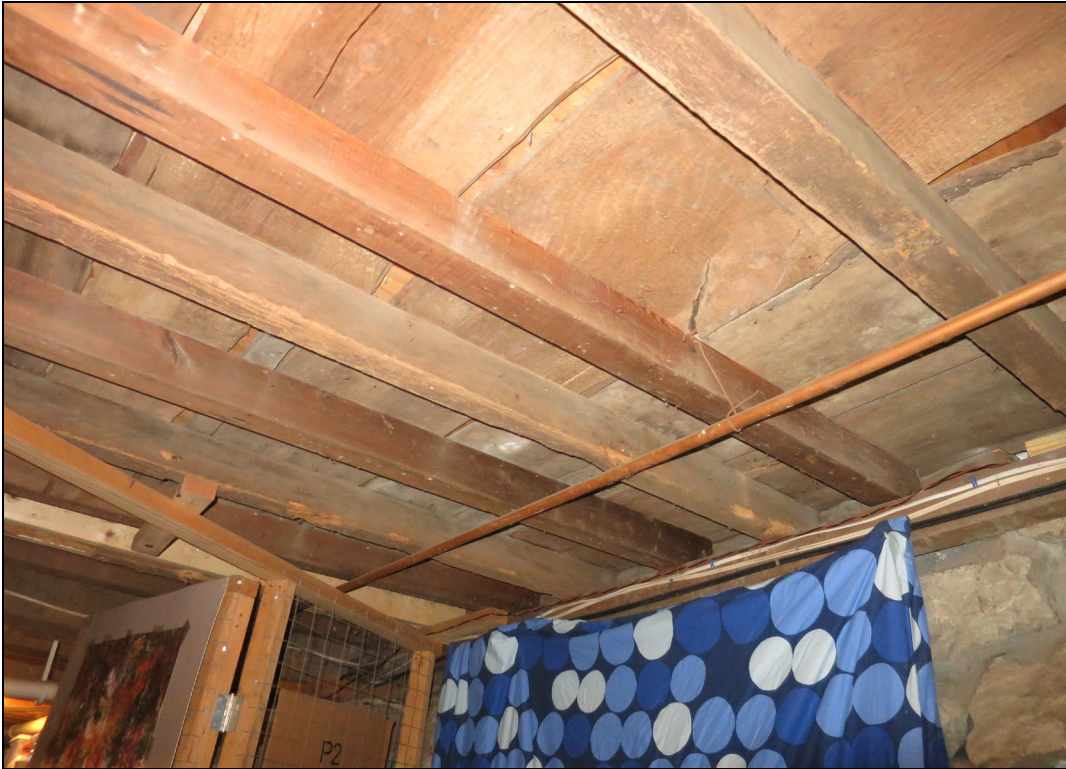
Basement, floor beams in ceiling.
