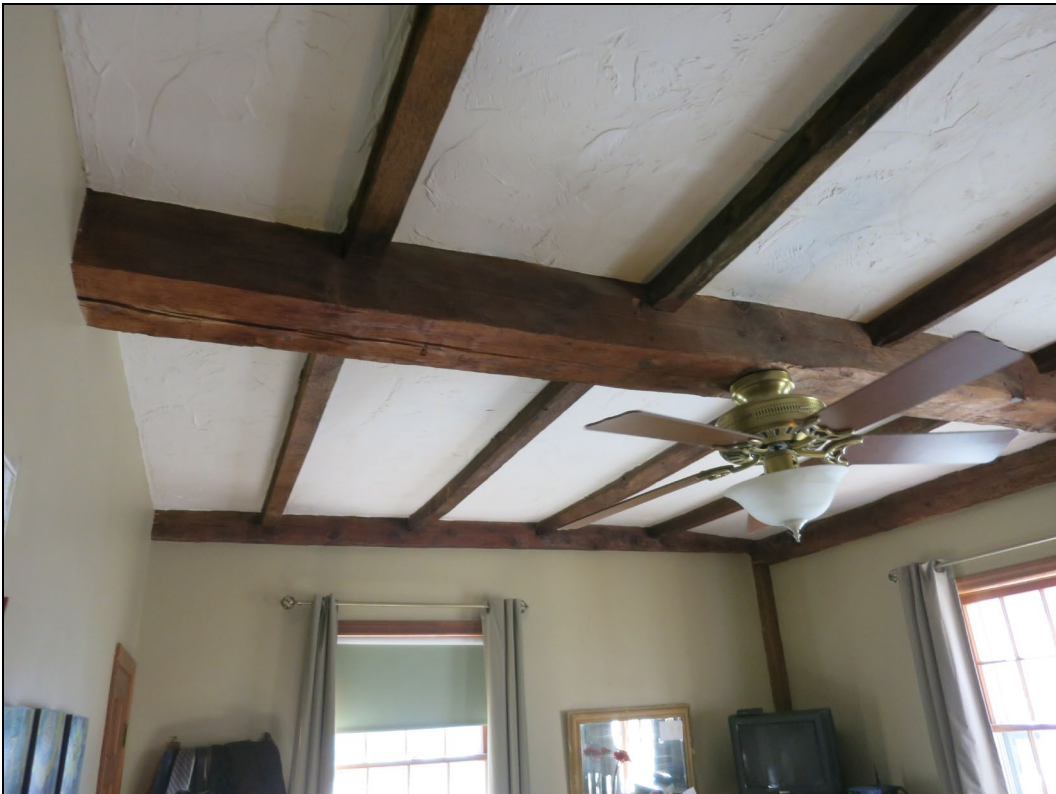
Second floor, south chamber looking south.
