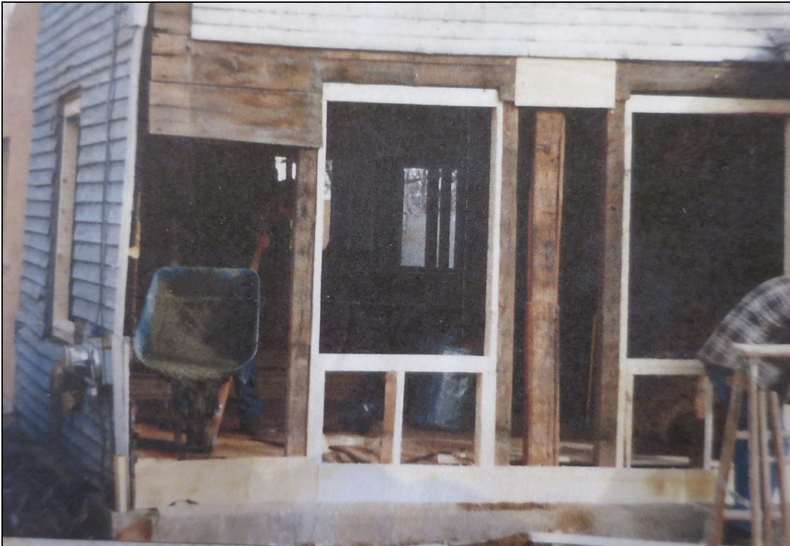
Detail of front wall showing renovation of window openings. Owner's collection.
