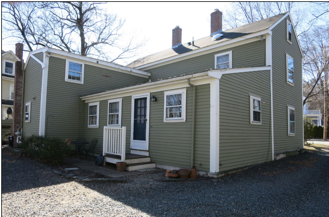
View from NE.
