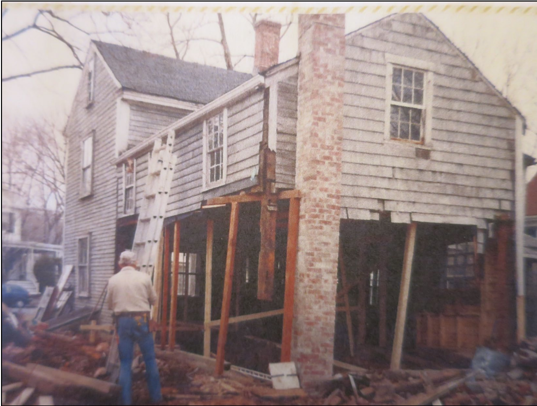
View of wing from SE during renovation. Owner's collection.
