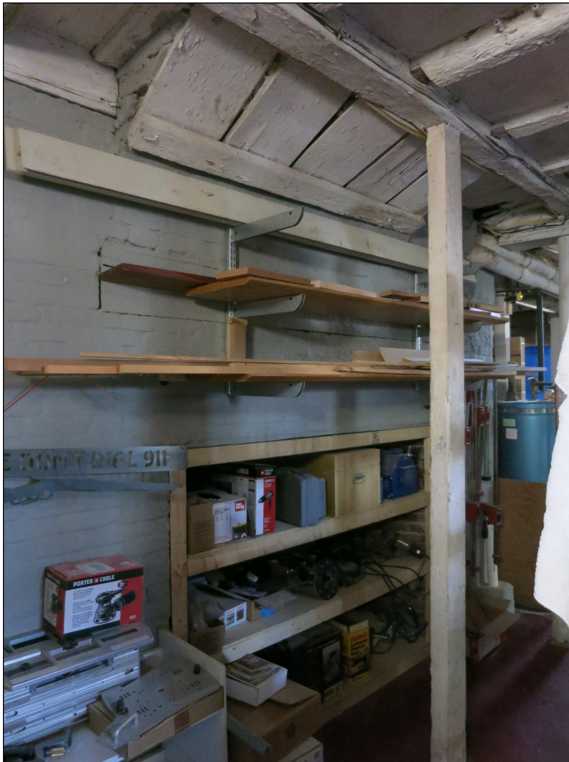
Photo 35: Basement, east side, fireplace(infilled with shelving) with Parlor hearth support above.
