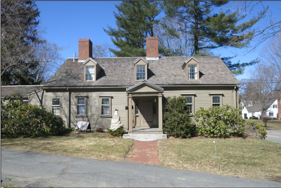
Photo 3: View from south.
