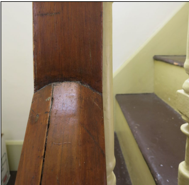
Photo 12: Detail of handrail showing two-part construction
