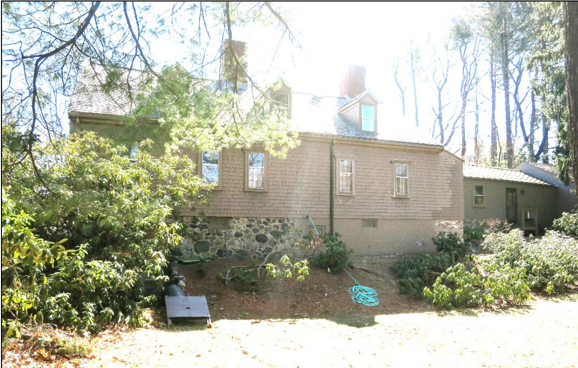
Photo 7: View from NE.
