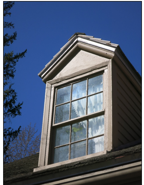
Photo 5: Detail of dormer.
