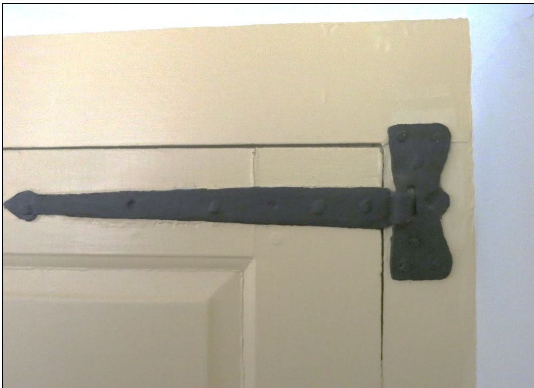
Photo 17: North Room, detail of "jimmer type" strap hinge on closet door.
