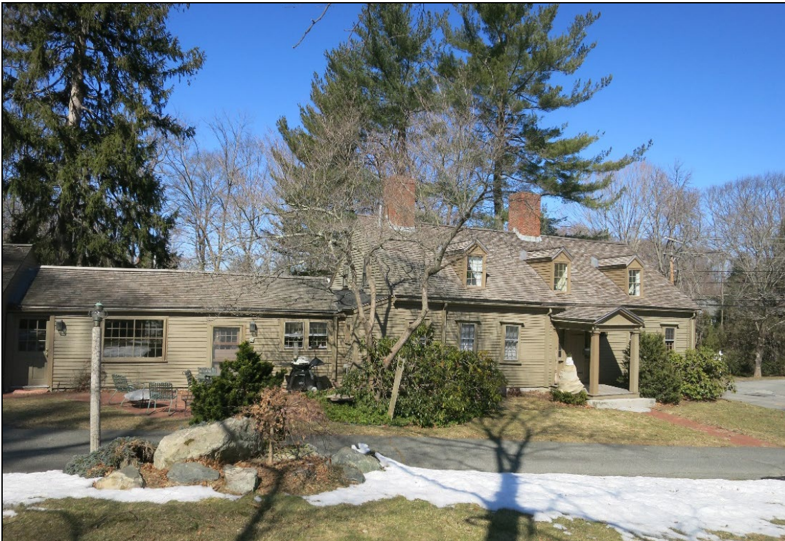
Photo 2: View from SW.
