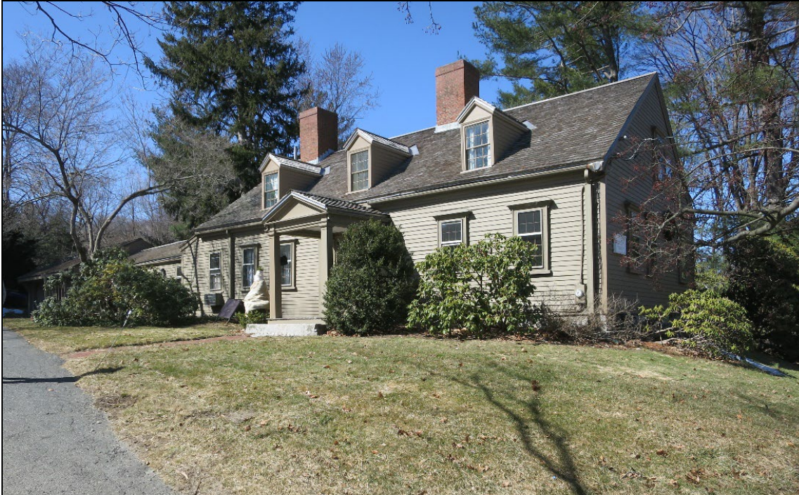
Photo 1: View from SE.
