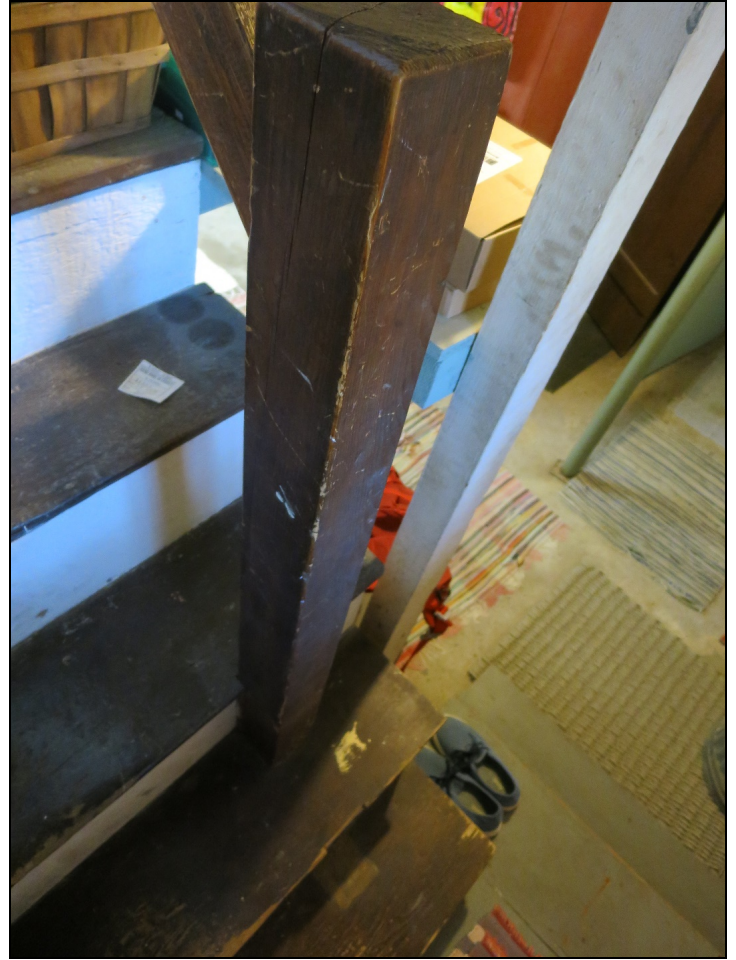
Photo 41: Post at bottom of basement stairs.
