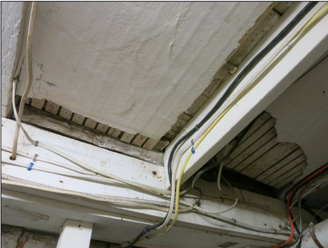
Photo 39: Detail of lath and plaster over whitewashed bottoms of floor boards.
