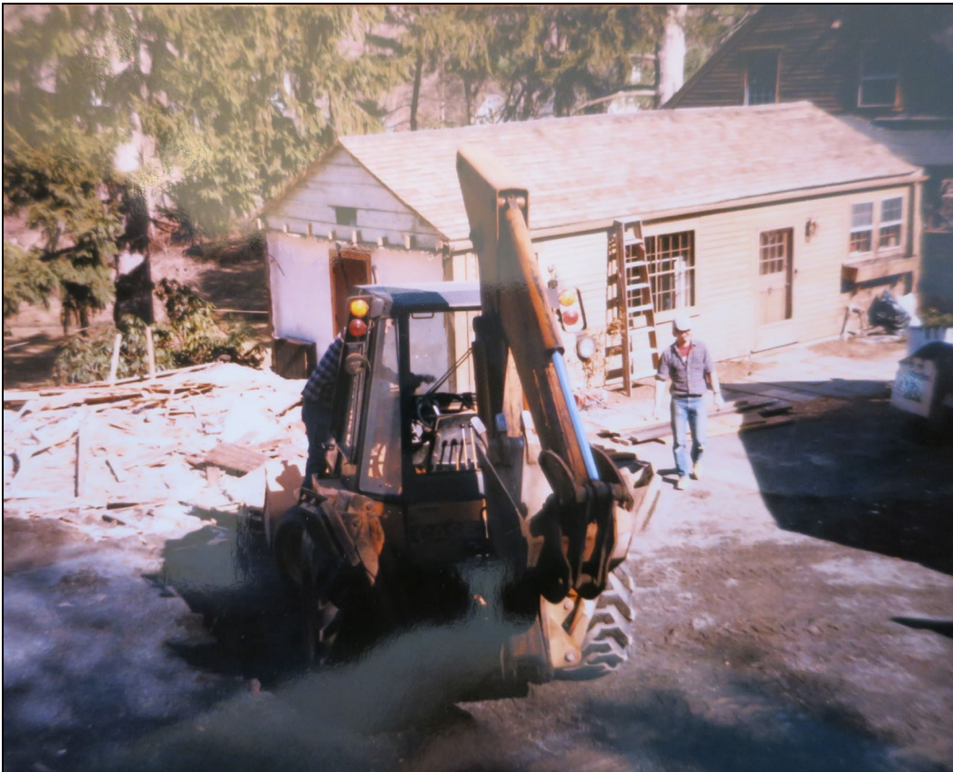
Fig.13: Construction of new attached garage, 1986. Owner's Collection.
