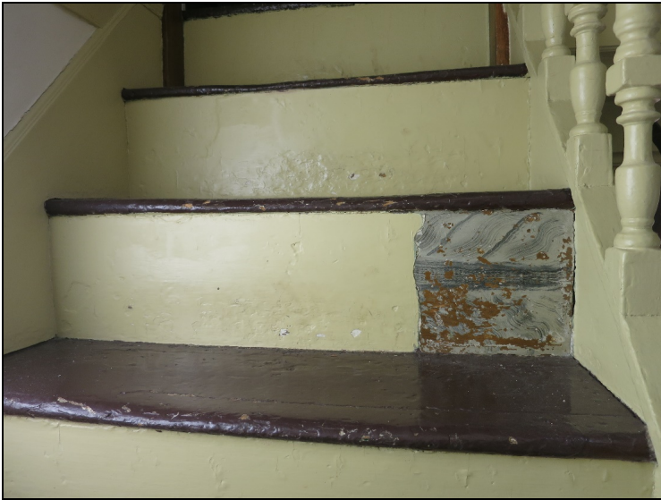
Photo 30: Detail of stairs showing exposed paint decoration.
