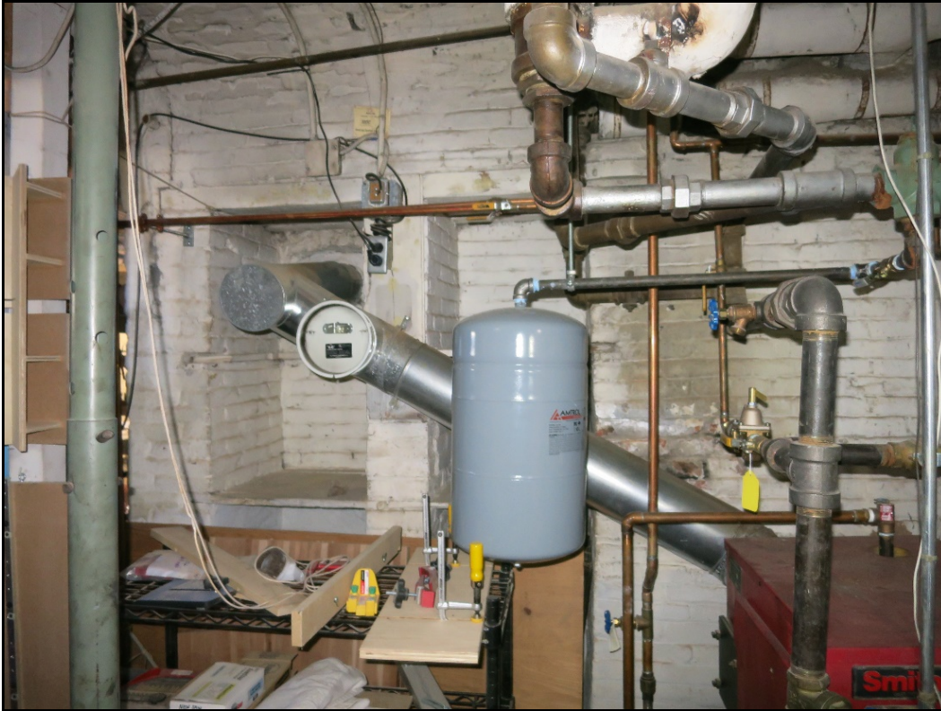
Photo 36: Basement, chimney base and brick arch supporting hearth in North Room.
