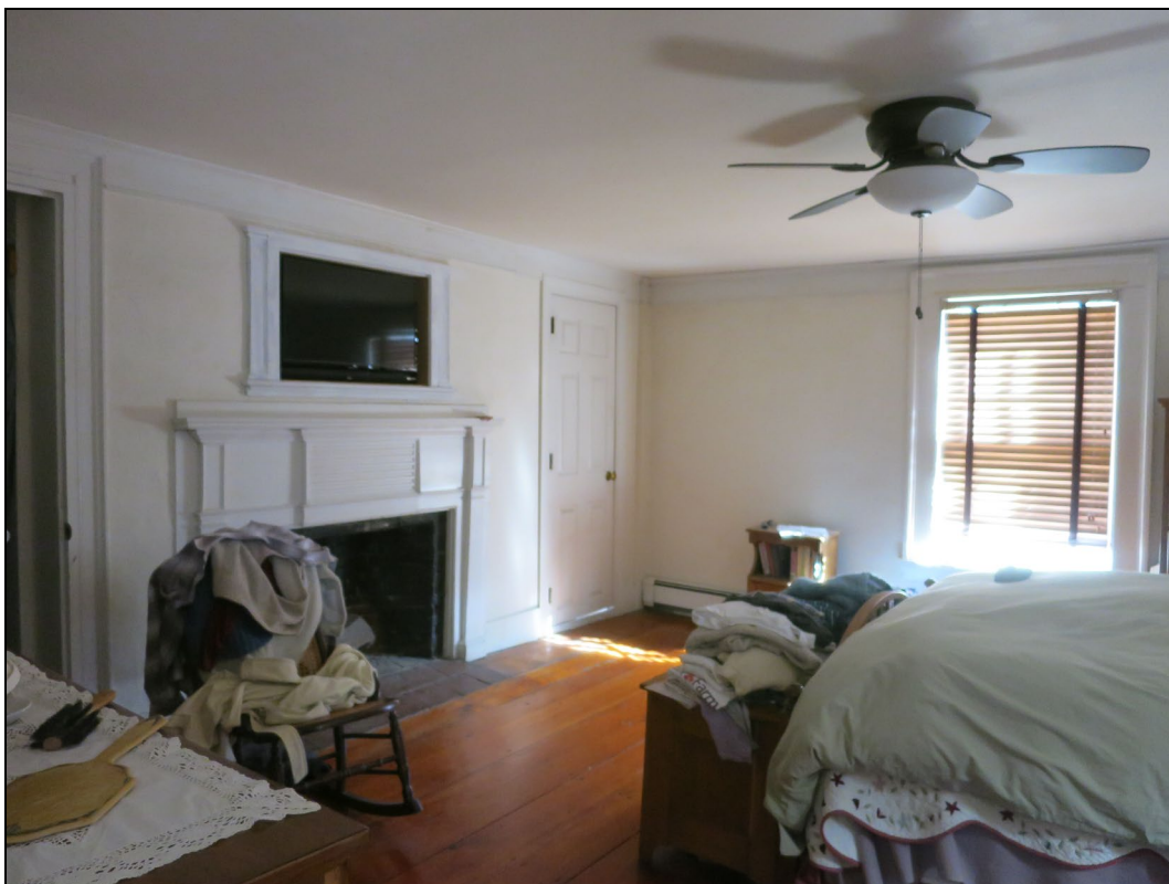
Second floor, SE front chamber looking NE.
