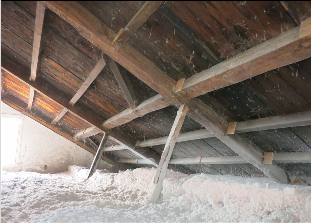
Attic, detail of roof framing, SE side.
