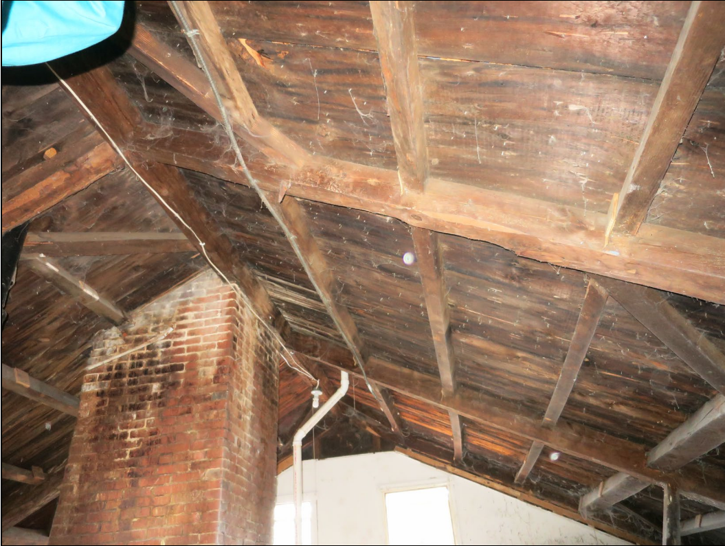
Attic, detail of roof framing showing ridge beam and chimney.
