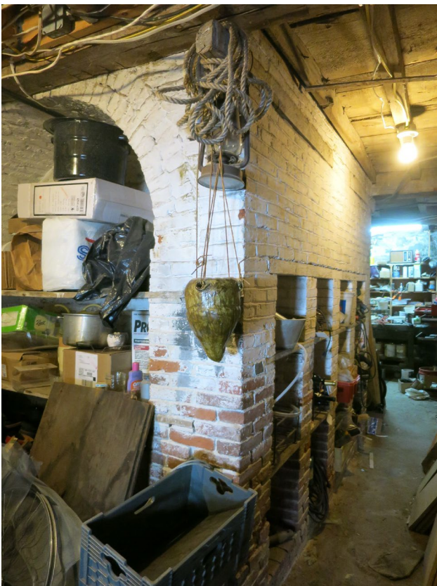
Basement, chimney base west side.
