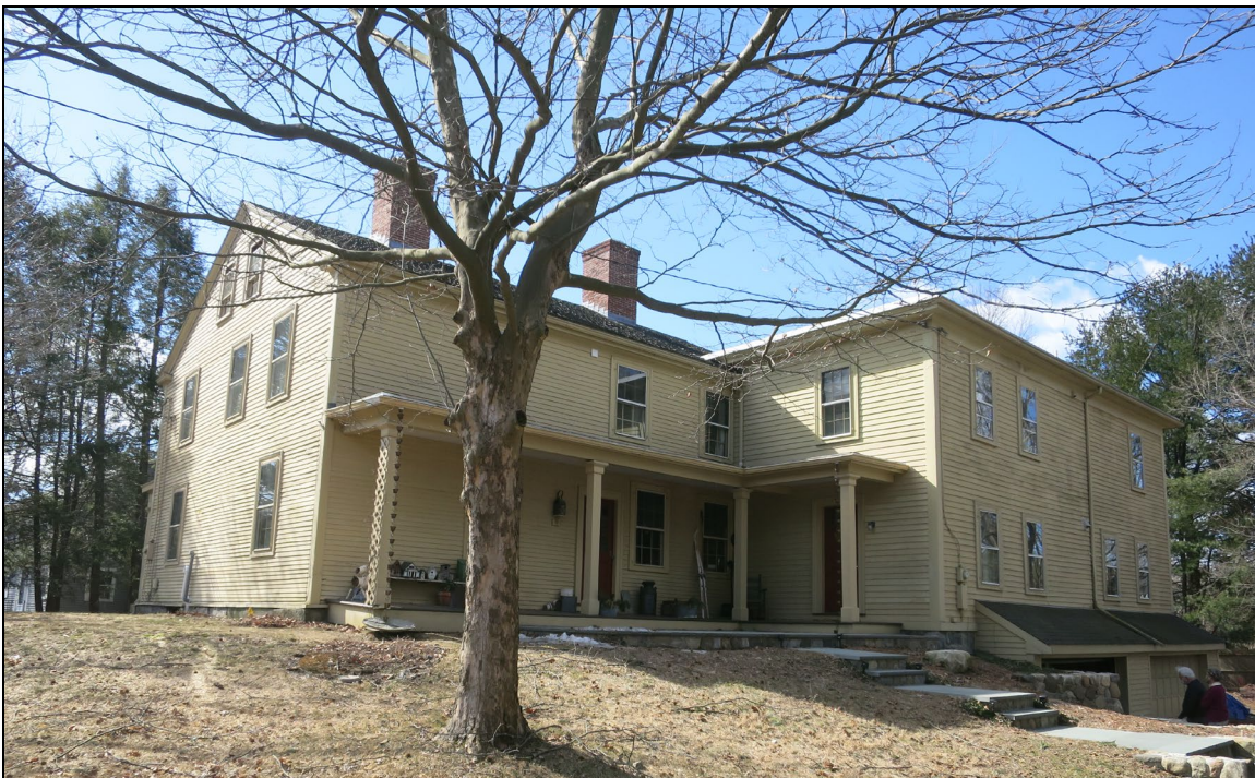
View from NE.
