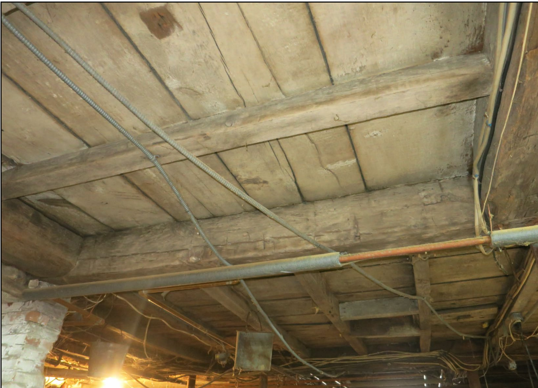
Basement, detail of floor framing.
