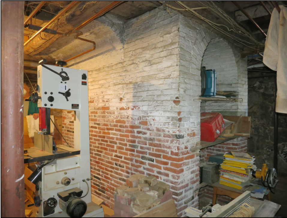
Basement, brick chimney base, east side.
