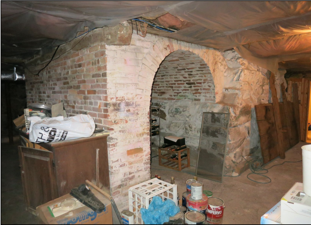
Basement, arched chimney base.
