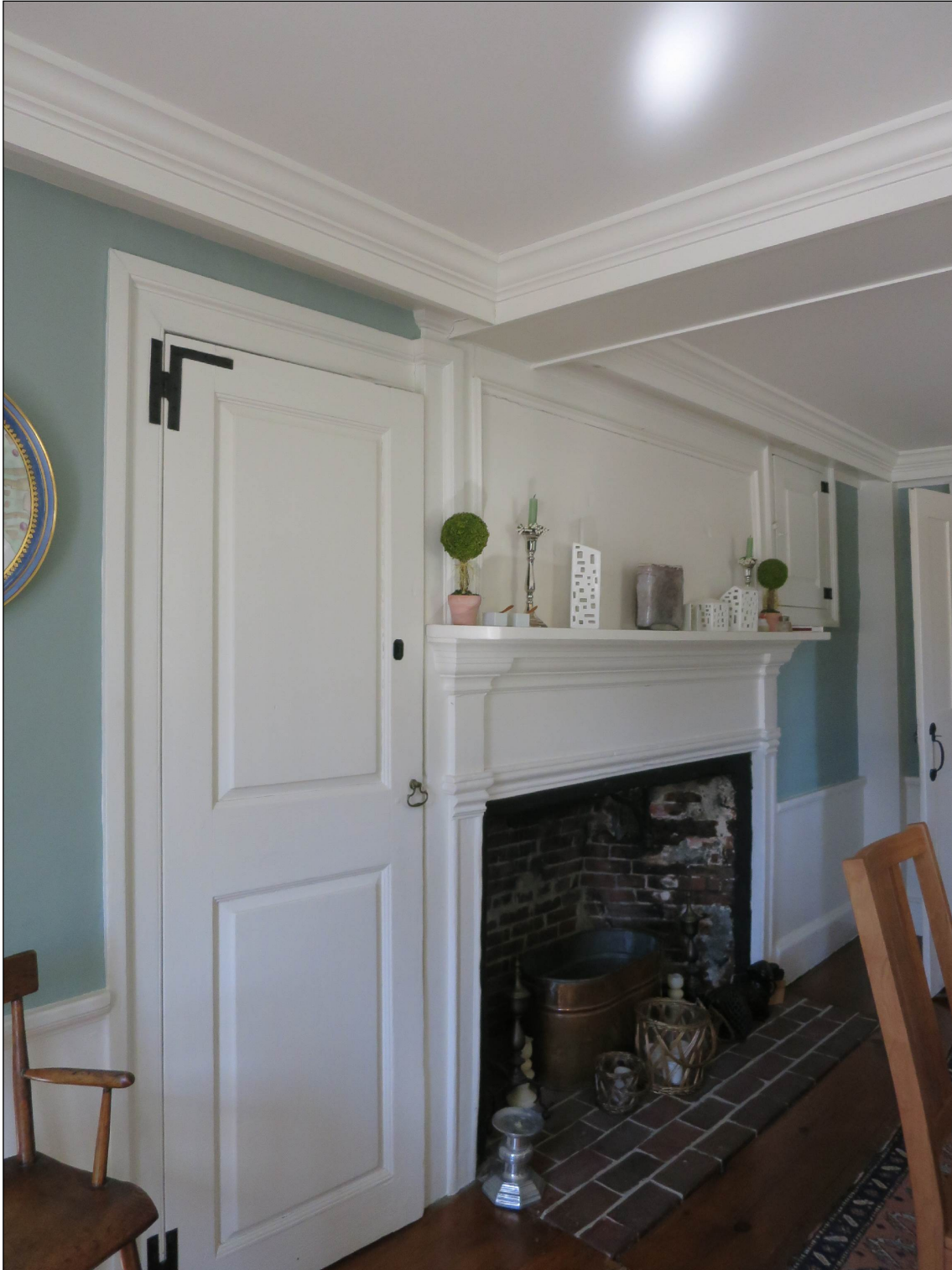
First floor, east parlor, chimney wall.
