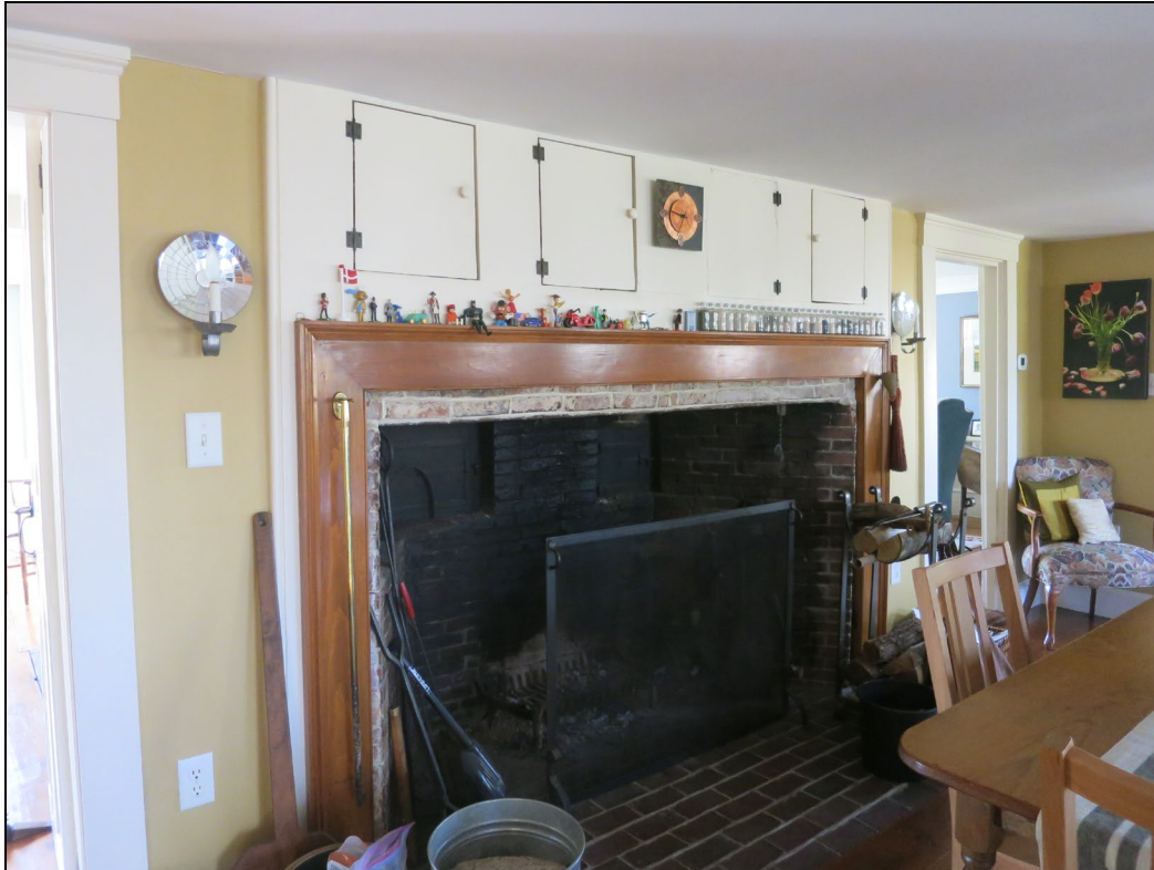
First floor, kitchen fireplace, paneling & mantel reconstructed.
