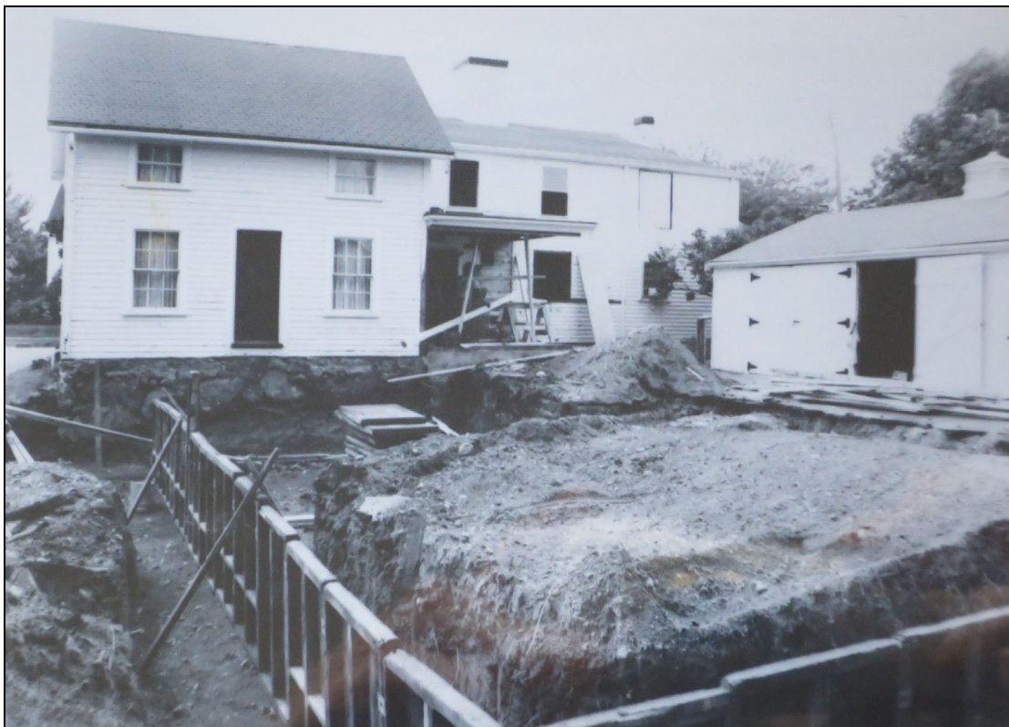
Excavation for addition, ca. 1979. Owners' collection.
