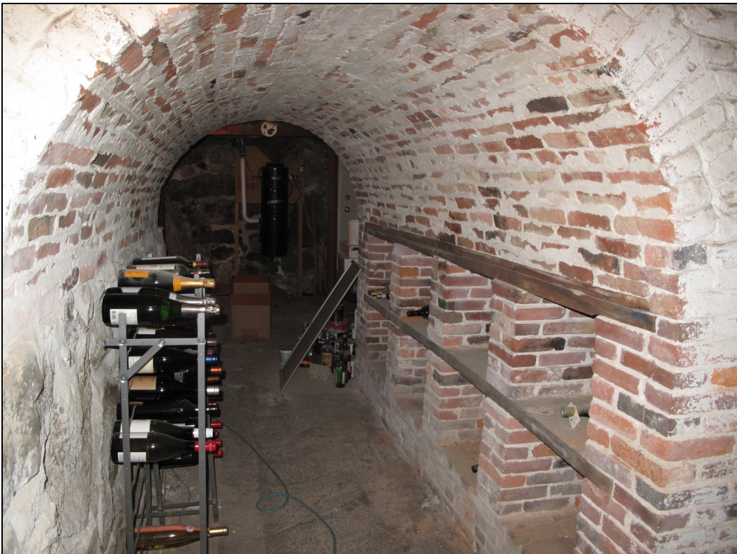
Basement, interior of chimney base arch with shelving.
