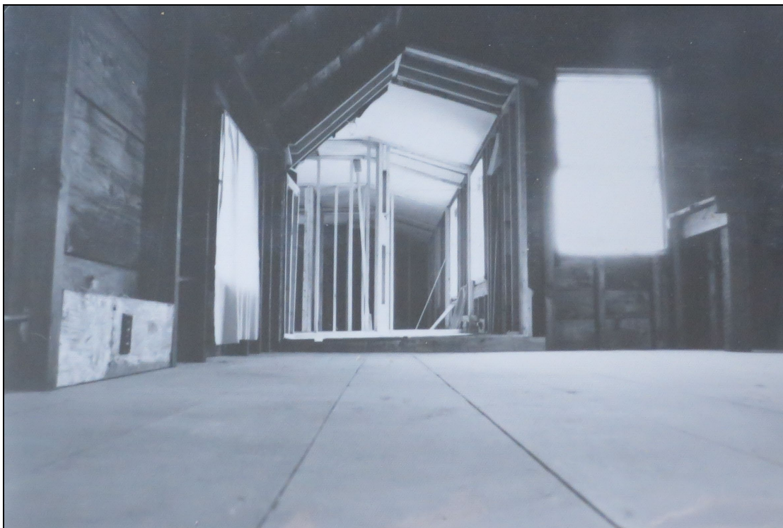
Renovation of upper story of lean-to, ca. 1979. Owners' collection.
