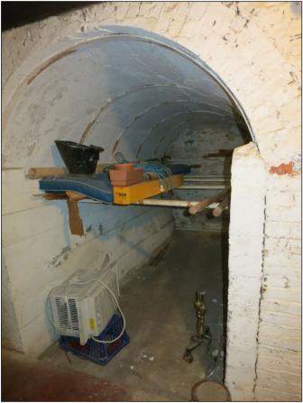
Basement of original house showing reinforced archway in base of center chimney.
