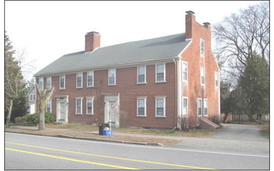
View from SW. Original ca. 1795 house/tavern with center chimney and five-bay façade on left with ca. 1810 addition with three-bay façade and brick end on right.
