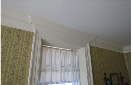
Detail of window, NW parlor, showing wall thickness to conceal posts and cornice.
